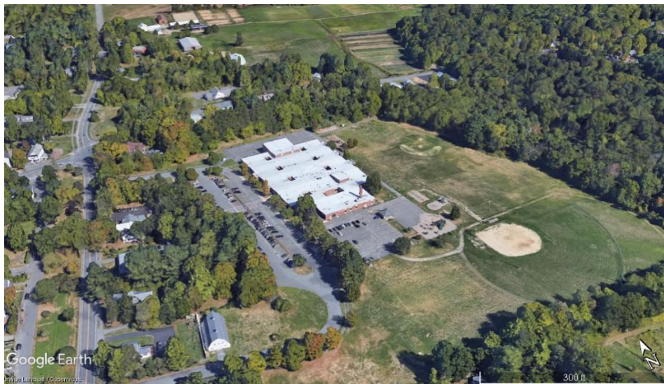
Figure 15. Fort River Elementary School Aerial
