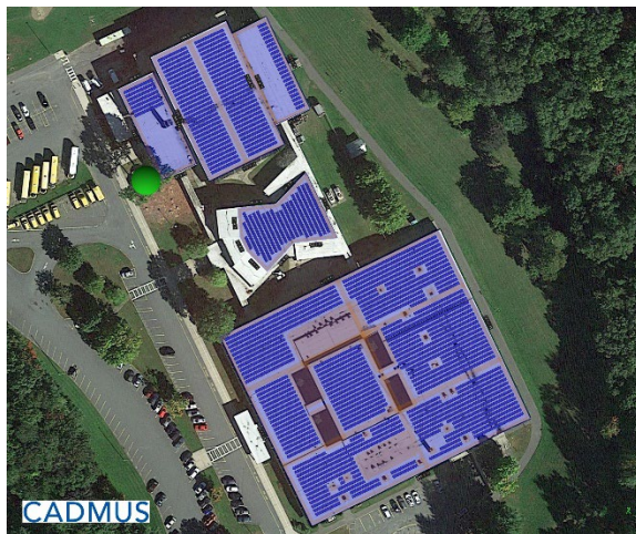
Middle School Roof
