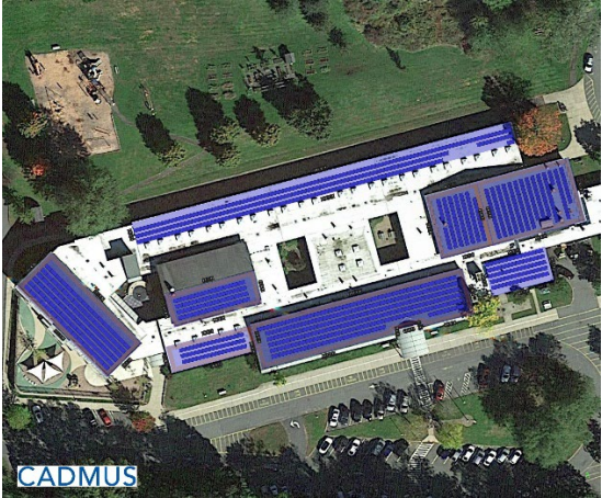
Crocker Farm Elementary Roof
