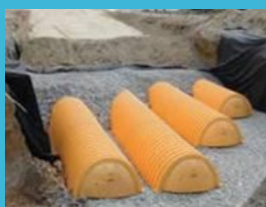
Devens Common underground infiltration systems
