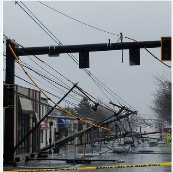
Arsenal Street experienced downed power lines during a storm in 2018.
